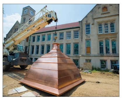
The new dome and weathervane, which replicate the original, were installed on the renovated clock tower in July 2011. The dome weighs approximately 700 pounds and is roughly 10 square feet at the base and 9 1/2 feet tall. The weathervane measures approximately 4 1/2 feet tall. The dome and vane are a copper finish and rest upon a copper cornice base.
